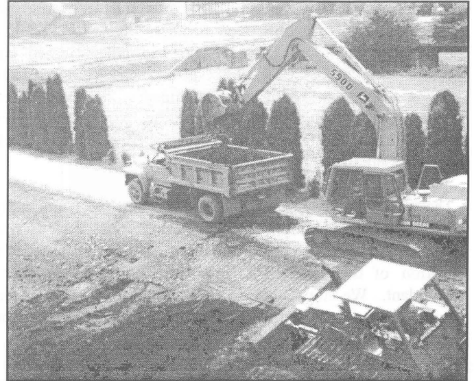
Heavy equipment 'dredges' the prism - Photograph courtesy Tom Perry
