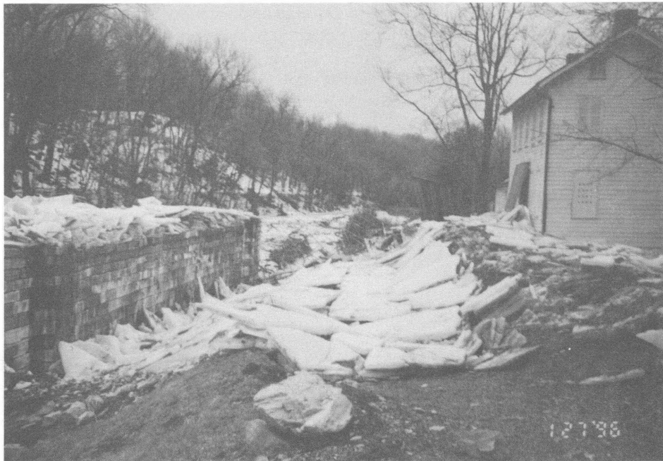
Lock 44 and Lockhouse sustained damage as a result of high water, ice, and debris. NPS photograph.
