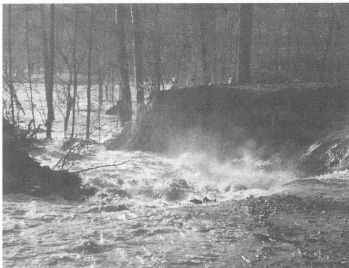
A break in the berm of the Canal occurred below Angler's Inn as a result of the January 1996 Flood. Could it have been avoided? Photograph courtesy NPS.
