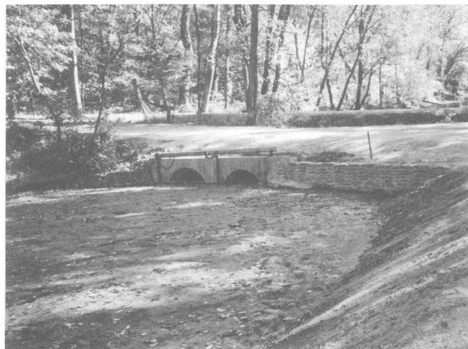
The earthen dike that contributed to the massive towpath break at Anglers Inn during the January 1996 flood will be removed and replaced by a bridge. This will allow the water in the canal to flow unimpeded and hopefully reduce the chance for future overtopping of the towpath during floods. Completion is scheduled for March 1999.
