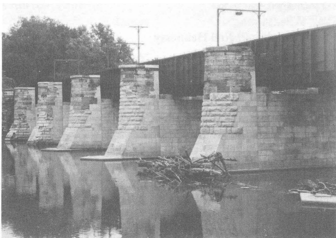
The Fox River Aqueduct, at Ottawa, is the longest on the Illinois & Michigan Canal. The prism trunk and towpath are supported by a series of piers. The aqueduct is maintained as part of the I&M Canal State Trail.
