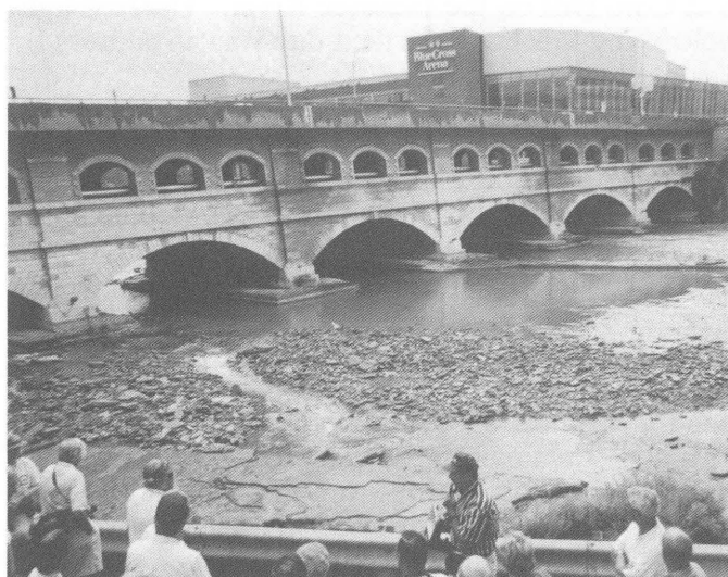
Conference delegates view the Genesee River Aqueduct in Rochester. When the barge canal replaced the old Erie Canal in 1918, the aqueduct was converted to a street bridge and is still in use.
