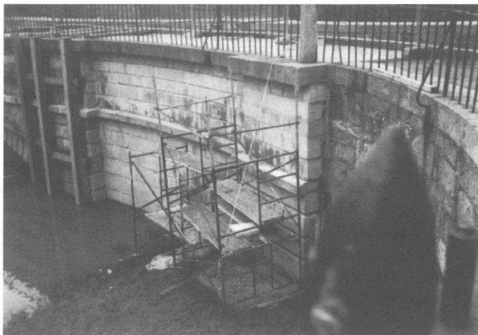
Scaffolding for Monocacy Aqueduct stabilization
