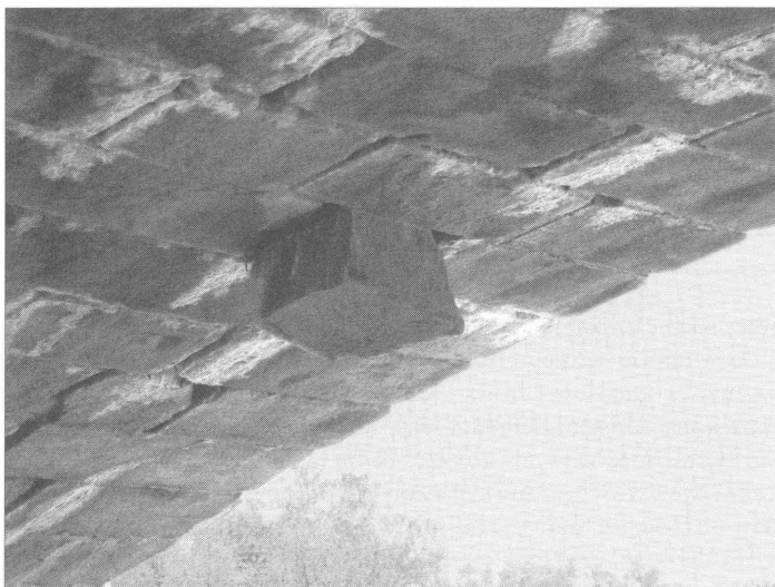
Over many years, the protruding stone shown above gradually moved out of line with the underside of the arch, and it has been allowed to remain in that position. The objective of Park Service engineers was to stabilize the aqueduct and to approximate its original appearance, but not to erase all visual effects of aging.
