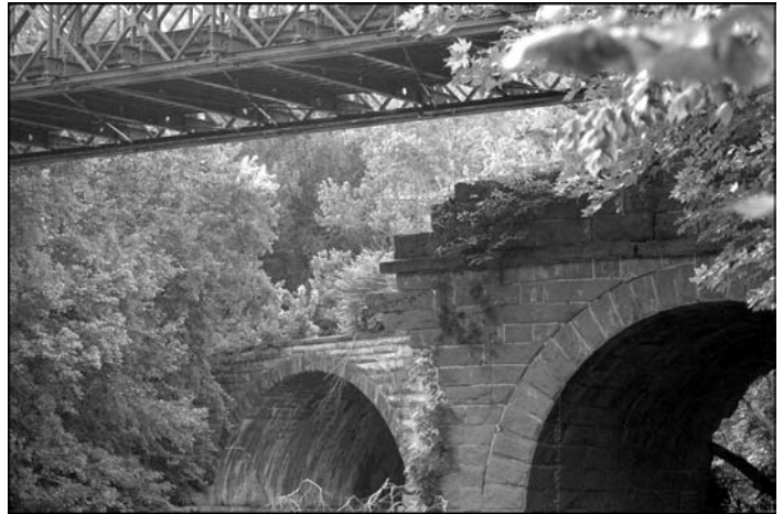
In the image above, the south side of Catoctin Aqueduct's east arch is shown in the foreground at right. The adjacent intact stone railroad bridge is in the background center. The military steel frame "towpath" bridge is shown at top. Photo by George Lewis, August 15, 2005.
