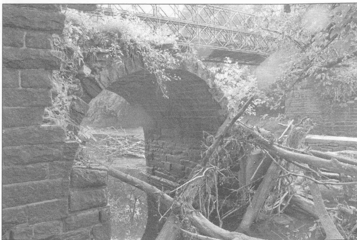
Catoctin Aqueduct: foreground, the fragile, debris-burdened up-creek side of the endangered east arch; background, the "temporary" Bailey bridge spanning the collapsed parts of the aqueduct, and the west wing wall and abutment. Photo: George Lewis
