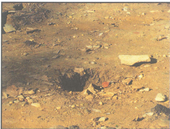
One of several small potholes on the canal floor next to breach. Photo by editor
