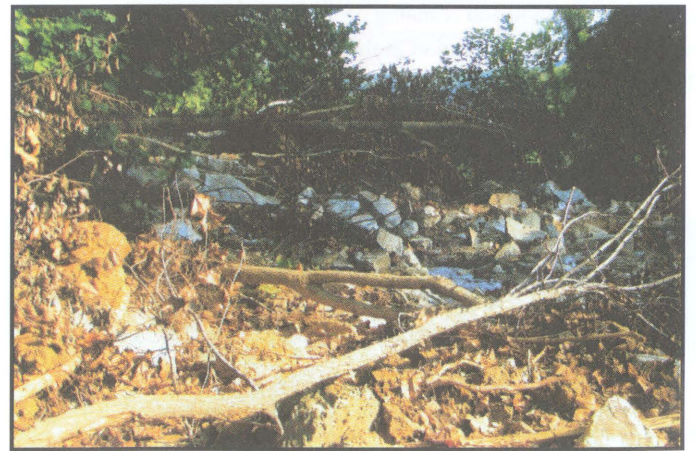
Debris & embankment stones scattered below the breach Photo by editor
