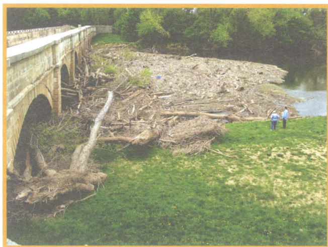
Flood-borne driftwood piled up against the Monocacy Aqueduct (April 18, 2010)
