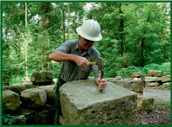
A lot of stones are being cut and dressed for placement in rebuilding the Catoctin Photo by George Lewis
