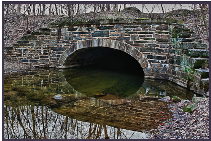
Culverts are crucial to canal integrity. Works of masonry craftsmanship, they come in all sizes and shapes on the C&O. See page 17.
