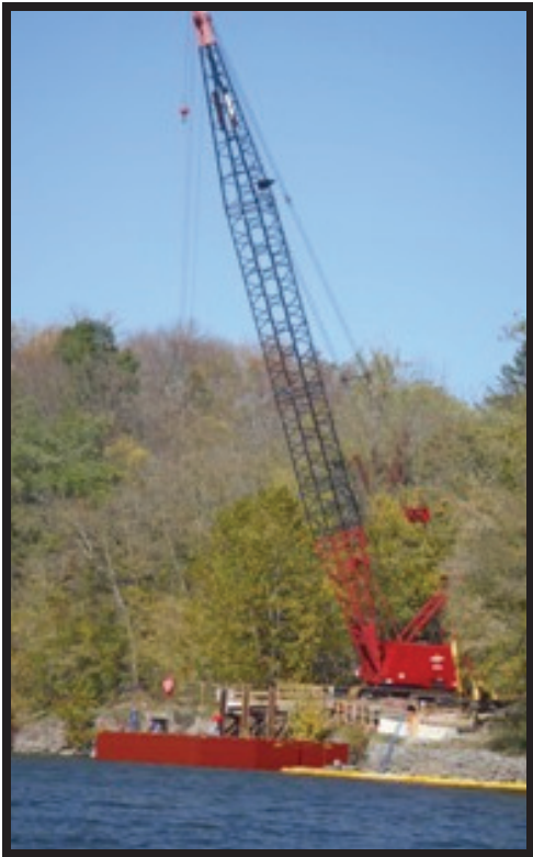
Crane at 160 ton capacity does heavy lifting re-building the towpath at Big Slackwater. See page five. Photo Courtesy of the NPS
