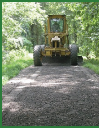
The Grader grades and levels
