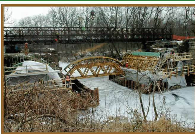
Restoring the Catoctin Aqueduct: Steel arch forms (above) are used in rebuilding the long central arch to close the gap left by the structure's collapse 38 years ago in a flash flood. See article and photos by George Lewis on the progress of the restoration on pages 3-4.
