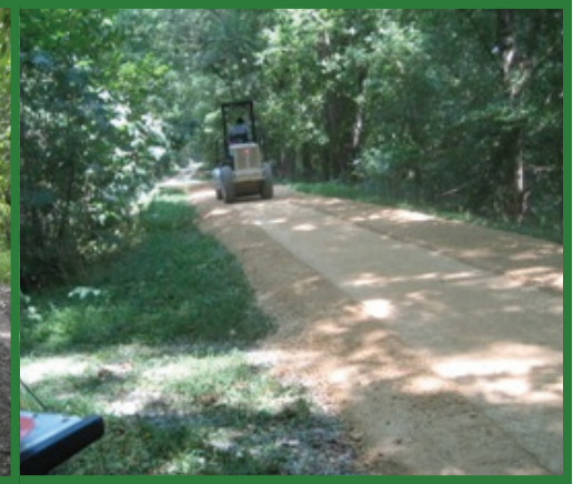
The Power Roller makes surface firm & smooth
