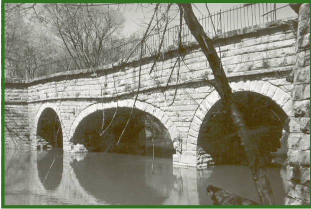
Aqueduct Weakens - Swayback in Middle Arch
