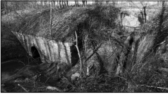
Culvert 86 and erosion - Photo by Doug Zveare
