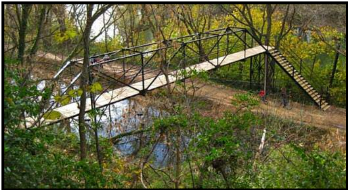
The Sycamore Island Bridge is a steel-girdered through-truss pedestrian bridge crossing the C&O Canal at mile 6.46. Built over a hundred years ago this picturesque bridge gave Sycamore Island Club members access to the towpath and Sycamore Island. The bridge's 20-foot height left room for canal boats to pass under it. The C&O Canal NHP's skilled maintenance staff recently restored the bridge to prime condition rust-proofing and painting the structure, laying down new planking and rebuilding the stairway down to the towpath. Photo courtesy of Joe Hage, Sycamore Island Caretaker
