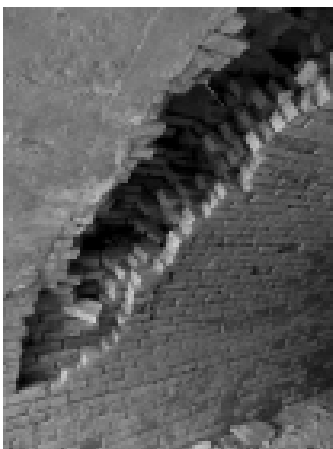
Brick damage in Culvert 208
