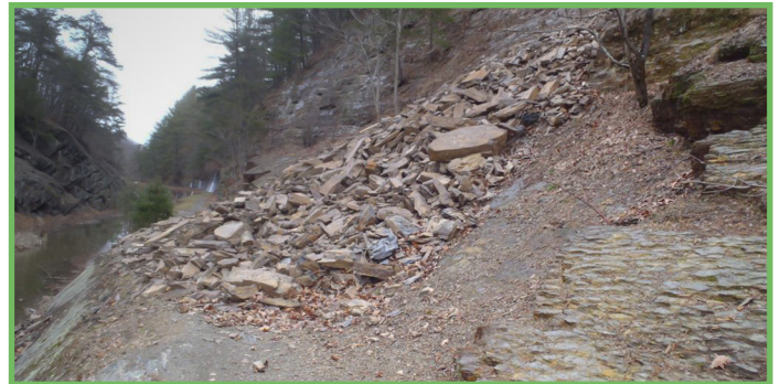
Rockslide blockage of the towpath below the tunnel
