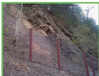
Left - The reopened towpath near mile marker 155. Right - The rock fall protection fencing that was installed to impede future rock slides. Photos courtesy of www.cocanal.com
