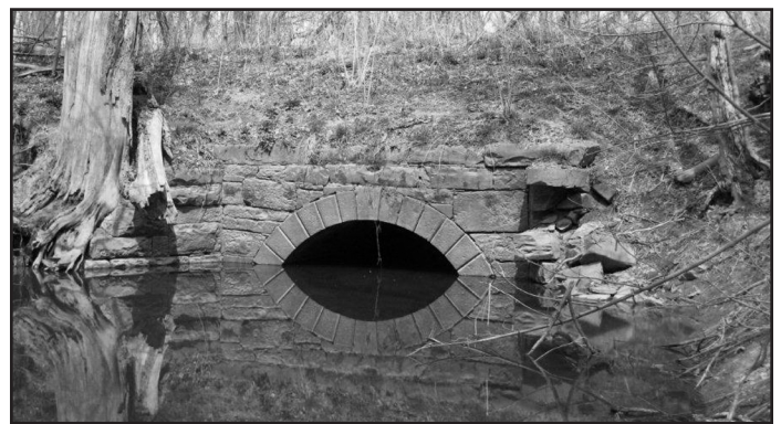
Culvert 42 (Note degraded downstream wing wall) – Photo by Pat Hopson
