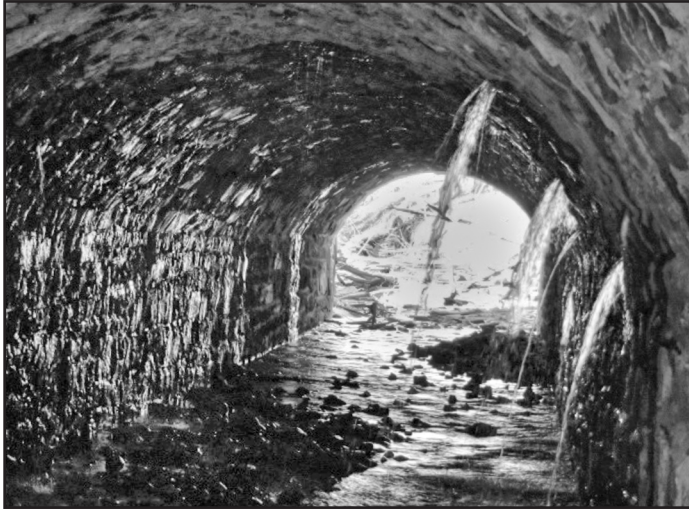
Water flowing into Culvert 185 – Photo by Paul Petkus
