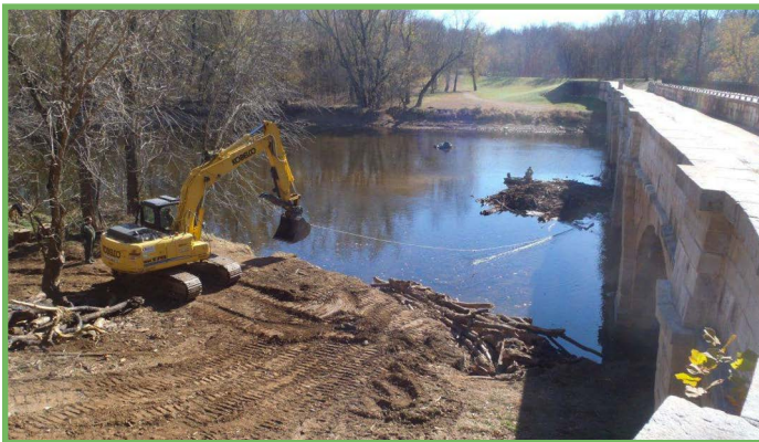
Left – The NPS uses heavy equipment to loosen and pull logs away from the 5th and 6th arches of the Monocacy Aqueduct. Right – one of the logs is dragged to the river edge. Photos courtesy of the NPS, C&O Canal NHP.
