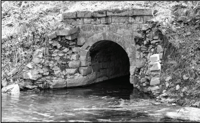
Culvert 100 continues to degrade, and has now lost both wing walls. Photo by Steve Dean
