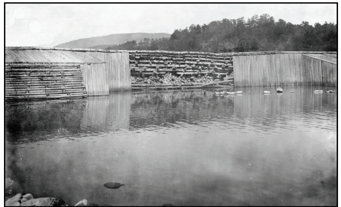
Dam 6 rubble construction – Photo courtesy of the NPS, C&O Canal NHP
