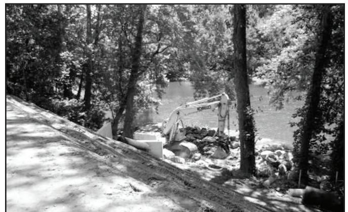
Below - The finishing touches on the culvert outflow to the river are shown in progress. Photos by Bob Mischler
