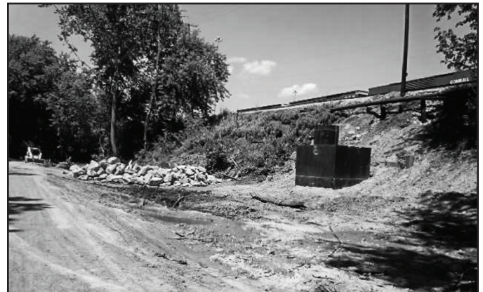
Above - The deep hole in the prism at the site of the washout near Mile 181.2 is now filled in and a drain vault is in place.
