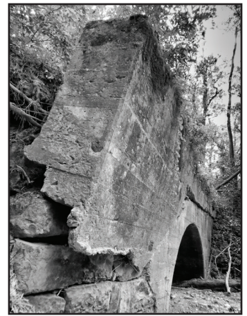
The concrete placed over the berm abutment of Culvert 208 is starting to fall off. Photo by Paul Petkus
