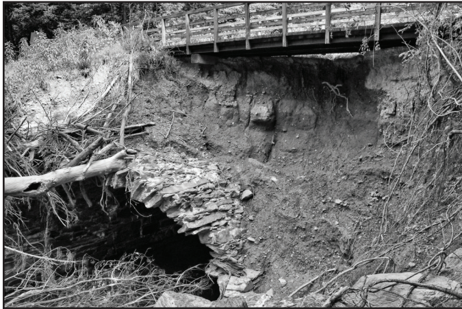
Flood damage over Culvert 82. The wooden walkway at the top of the photograph carries the towpath over the culvert arch. Photo by Doug Zveare
