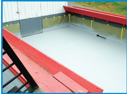
The Cumberland is an outdoor static display at Canal Place. This picture shows new plywood decking coated with Line-X waterproofing material. Photo by Rita Knox, NPS
