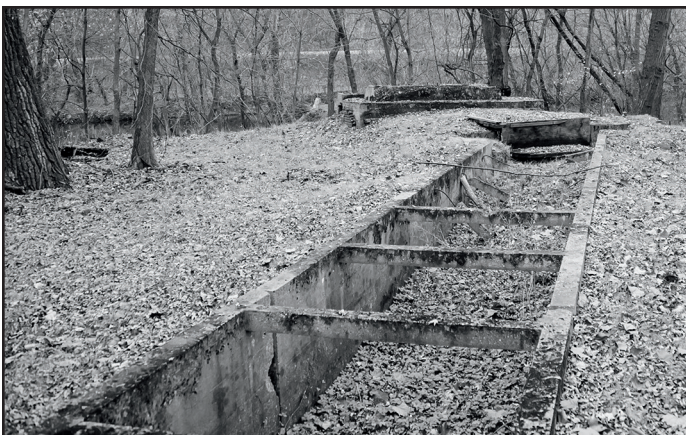
This flume allowed water pumped from the river to flow into the canal. The pump was located on the foundation in the background. The pump was required because Dam 7 was never built.
