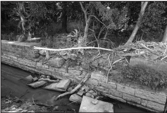
Fallen stone work and debris at the Goose Creek river lock. Photo by Pat Hopson
