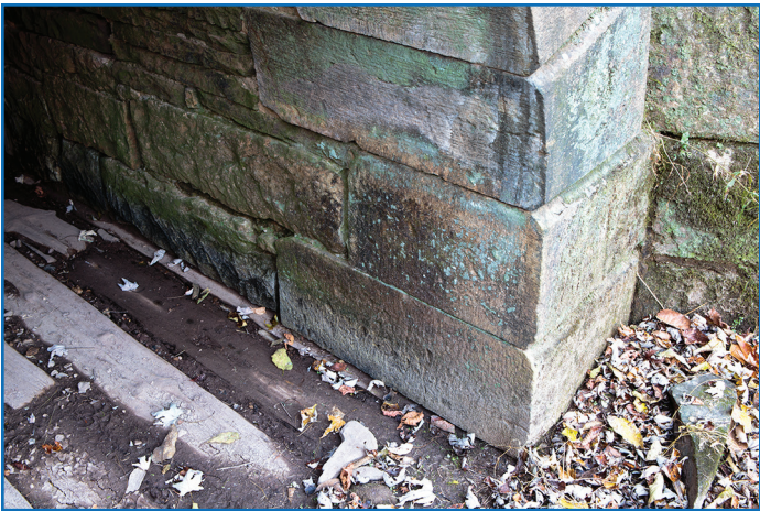
This detail of the base of Culvert 202 illustrates how some culverts are built on wooden foundations. The wood is often well preserved because it is typically under water. Low water levels of many streams in the fall of 2016 allowed close observation of the culvert foundations. Some wooden base culverts have degraded over time. Culvert 202 is in good condition and the wood is intact and solid. Contact Steve at editor@candocanal.org for further discussion of culverts. Photo by Steve Dean
