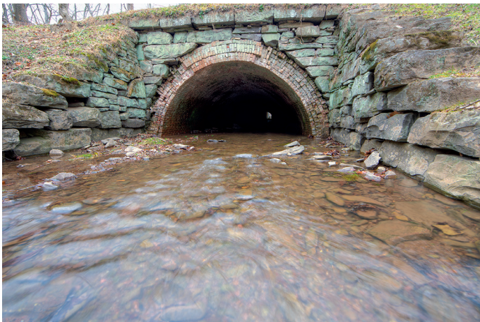
Culvert 215 is a well preserved culvert located just below Town Creek. The 16-foot brick arch and barrel have held up well and the wing walls of rough cut stone are intact. The culvert carries Big Run, which drains from Green Ridge. The downstream arch is shown here; the upstream end of the culvert is extended under the abandoned Western Maryland Railway and Md. Route 51. – Photo by Steve Dean
