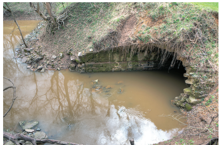
The wetlands restoration plan notes that Culvert 71, which spans Tuscarora Creek, requires repairs to protect the potential restoration of the surrounding wetlands area. Photo by Steve Dean
