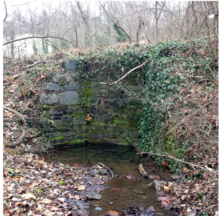
The silted outlet arch is below the water line in this image.
