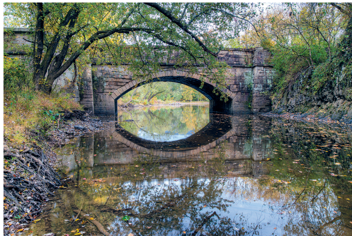
Fifteen Mile Creek (Mile 140.90) – This aqueduct is easily accessed and viewed in Little Orleans. It is in excellent condition, with both the towpath and berm walls intact.
