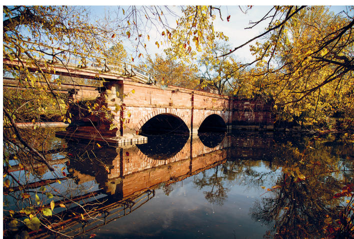
Seneca Creek (Mile 22.82) – This 3-arch aqueduct is combined with a lock and is made from Seneca stone. A 1971 flood washed out the upstream arch. With public support it may someday be restored.
