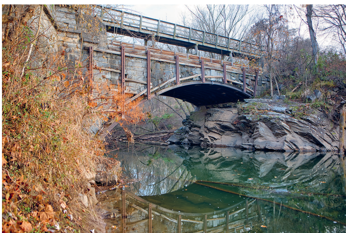
Tonoloway Creek (Mile 122.96) – Located in the canal town of Hancock, this aqueduct features an irregular arch that rests on a rocky ledge on the downstream side.
