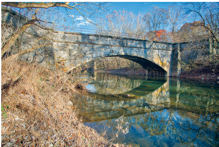
Licking Creek (Mile 116.30) – The first of the single-arch aqueducts is also the longest, with a 90-foot span. Concrete repairs have been required because of weak stones used in its construction.
