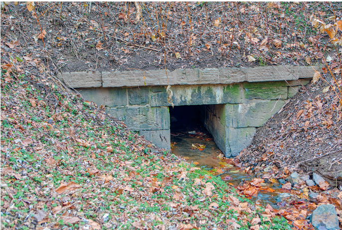
Culvert 175 is one of two existing box culverts on the canal. Also known as a "square drain," it is located at Mile 122.49 near Hancock. It measures 4 feet wide by 3 feet high. Box culverts were simple in design and well suited for small streams. Culvert 46 ½ is the other box culvert and is located near Whites Ferry. Nov. 13, 2017. Photo by Steve Dean
