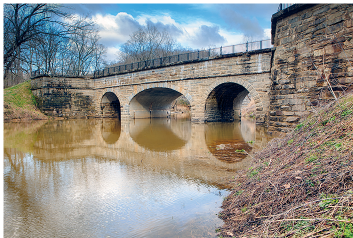
Catoctin Creek (Mile 51.53) – Two of this aqueduct's three arches collapsed in 1973. A restoration project was completed in 2011 and used many of the original stones
