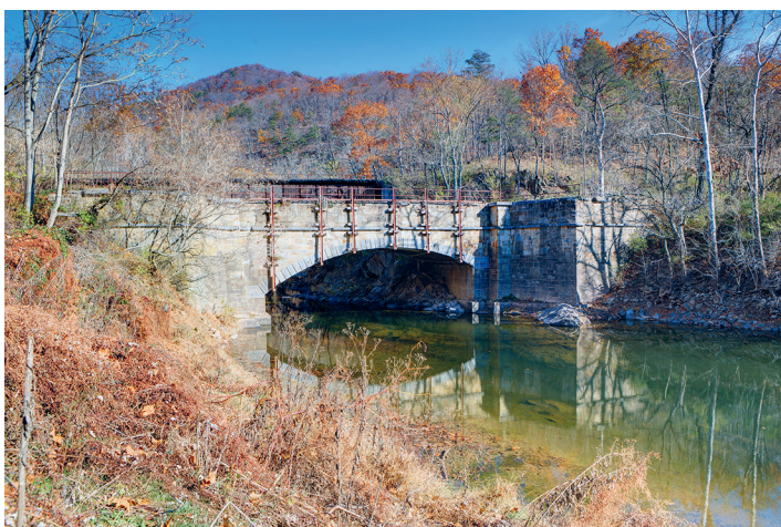
Sideling Hill Creek (Mile 136.56) – This aqueduct is located in a quiet area at the foot of Sideling Hill near Pearre. It features a 60-foot asymmetrical arch.
