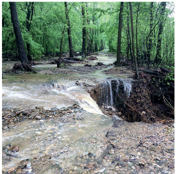
Towpath washout near Mile Marker 64
