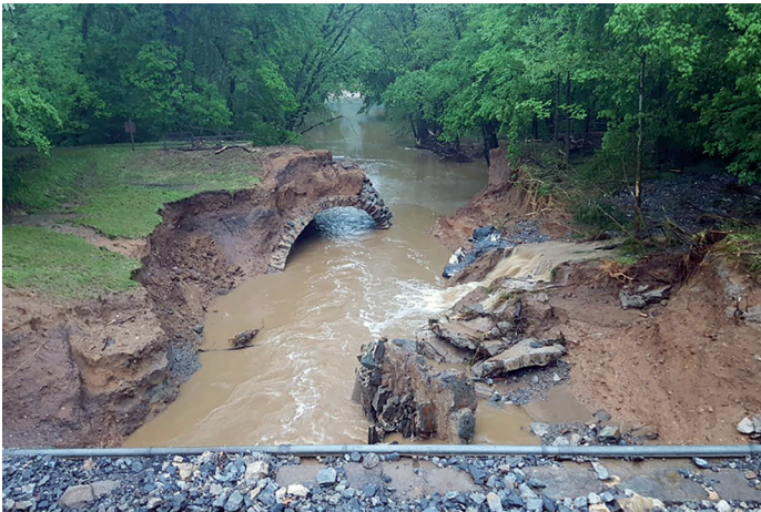
Another view of the towpath breach at Culvert 82 – All photos courtesy of the Chesapeake and Ohio Canal NHP, National Park Service
