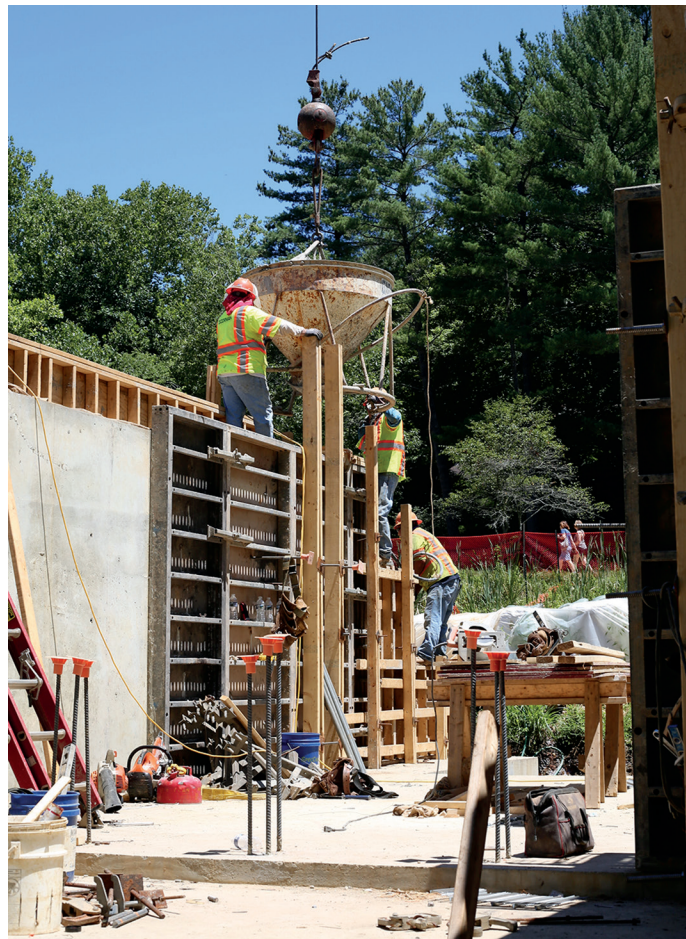
Construction workers pour concrete to form the walls of the Lock 20 waste weir replacement – Photo by Stephanie Spencer
