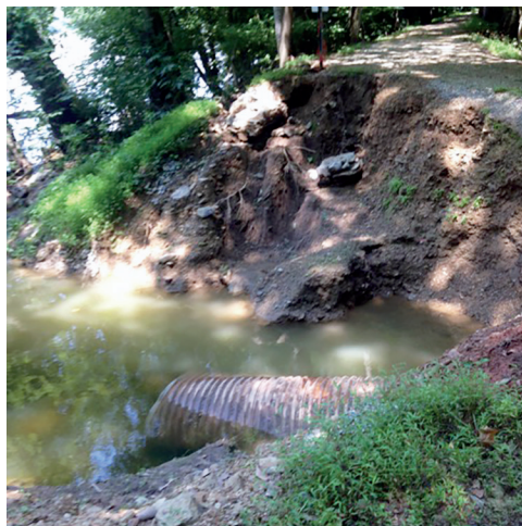
Culvert washout near Dargans Bend – Photo by Don Juran
