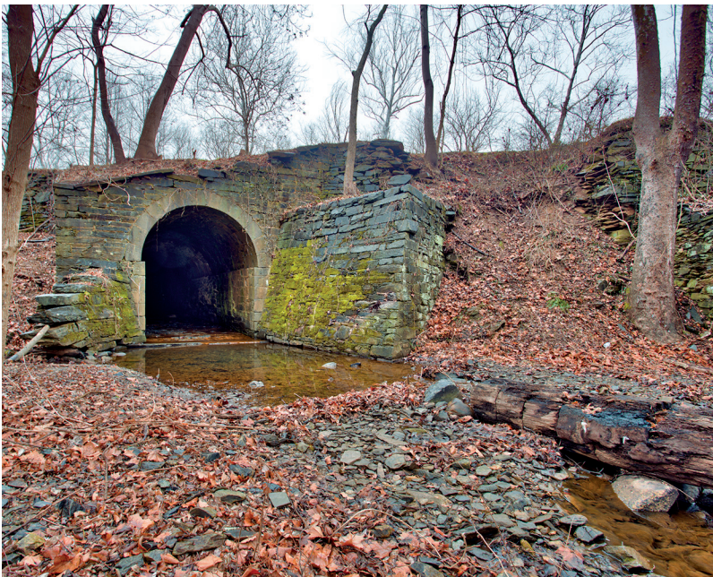
Rock Run Culvert (Mile 8.93). Note the retaining wall failure on the right – Photo by Steve Dean
