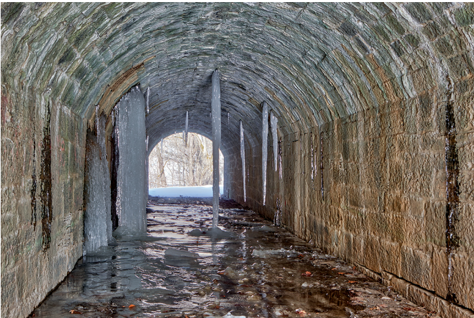
Culverts are often leaky, but we may not notice because there isn't always water in the prism over them. Culvert 142 at McCoys Ferry (Mile 110.42) is an active road culvert, but in February it was closed due to a significant formation of ice and a very slippery road surface. Photo by Steve Dean
