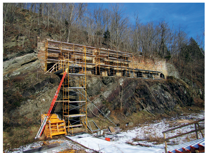
The kilns with the installed scaffolding
