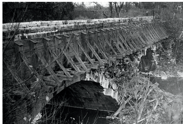
1920: Completed berm wall repairs with timber – Photo C&O Canal NHP, National Park Service
