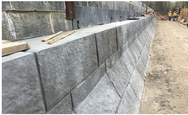
Above – The towpath side of the aqueduct, stamped to resemble stone
