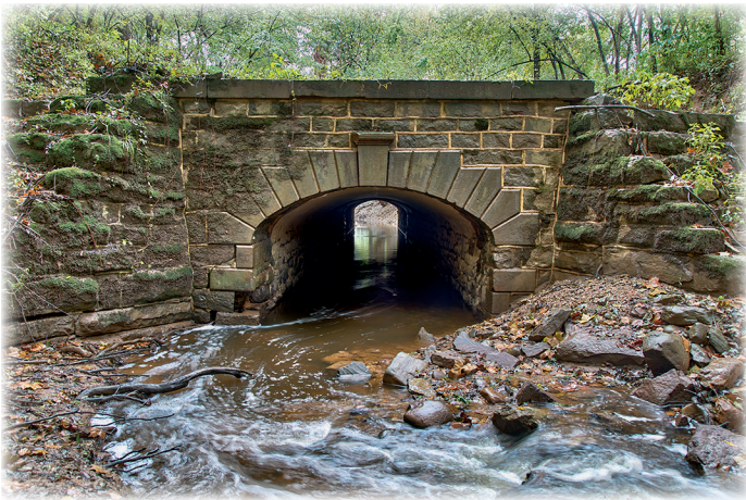
Culvert 49, at Mile 34.82, is known for the ornate stonework of its arch. Although an active stream now flows through, it may have once been a road culvert for Whites Ferry that has silted in. Photo by Steve Dean
