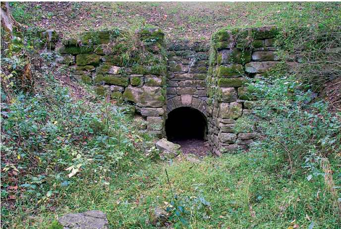
Culvert 135, at Mile 102.65, drains a generally active stream. The upstream arch, shown here during a dry spell in 2016, features a 6-foot span and high 90 degree wing walls. The downstream arch drains directly into the river. Photo by Steve Dean
