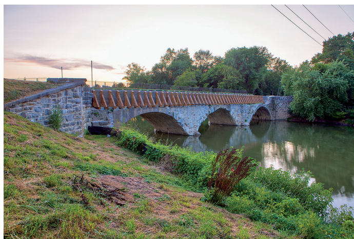
Above – The aqueduct berm wall is designed to appear as it did in the 1920s, with a wooden wall
