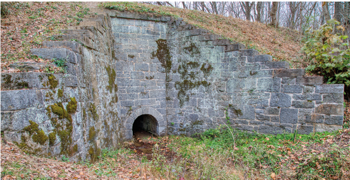
Culvert 141, at Mile 110.1, is easily viewed – one has to simply walk to the lower end of the McCoy's Ferry campground. It features a distinctive 15-foot high parapet that is similar in design to Culvert 144 about 3/4 mile upstream. This 4-foot arch stream culvert was originally intended to be a rectangular box type until the Canal Company opted for a uniform design of semi-circular arches on smaller culverts. Photo by Steve Dean
