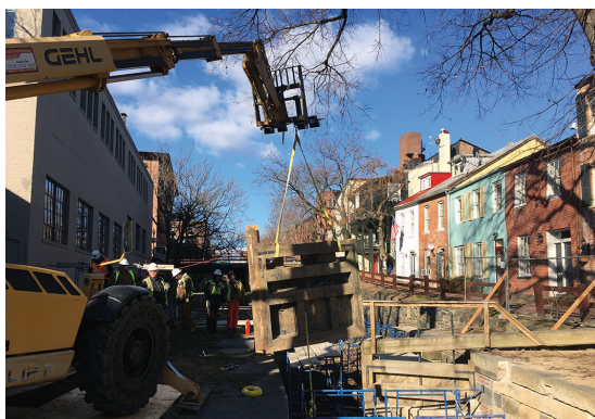
Top – The exposed timber foundation of Lock 3 Middle – Pallets of cataloged stones from Lock 3 Bottom – Removal of the deteriorating gates at Lock 4 Photos by Joe Reed, C&O Canal NHP Civil Engineer
