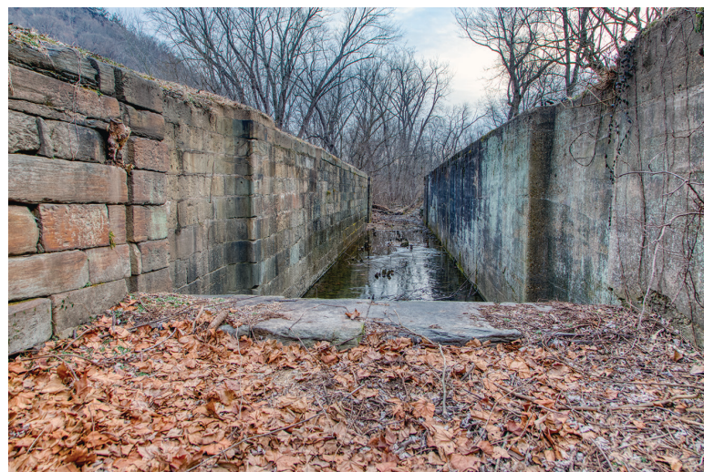
Lock 31 walls from the upstream end of the lock, with the concrete-faced shaved stone towpath side wall – Photo by Steve Dean
