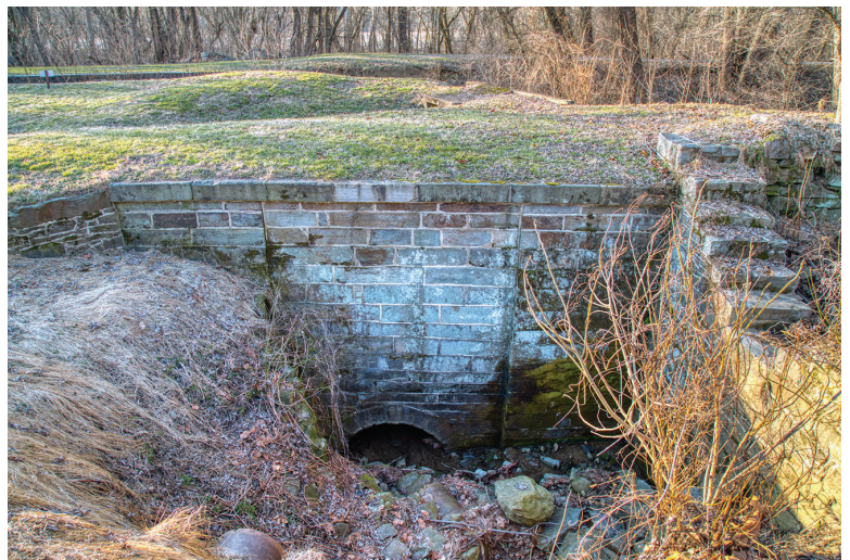
The berm side of the culvert under Lock 31 in 2016, showing alignment with the upstream section of the lock – Photo by Steve Dean
