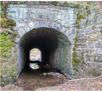
Culvert 150, at Mile 140.4 in the Ernstville area, is a 12 foot span road culvert that once provided river and ferry access to Cherry Run. It now carries a steady stream from the Ernstville area. The culvert features extensive wing walls on the towpath side. Photos by Steve Dean
