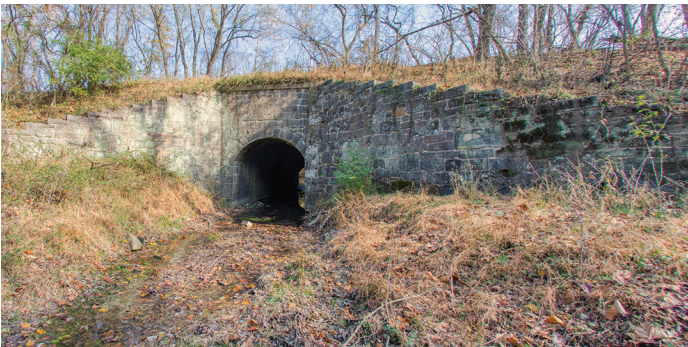
Culvert 150, at Mile 140.4 in the Ernstville area, is a 12 foot span road culvert that once provided river and ferry access to Cherry Run. It now carries a steady stream from the Ernstville area. The culvert features extensive wing walls on the towpath side. Photos by Steve Dean
