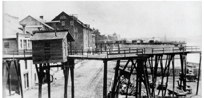
The Georgetown trestles allowed coal to be transported from the canal to the waterfront, but then it had to be lowered into holds of the ships or dumped down – which broke the coal up badly. Image courtesy of the C&O Canal National Historical Park, National Park Service
