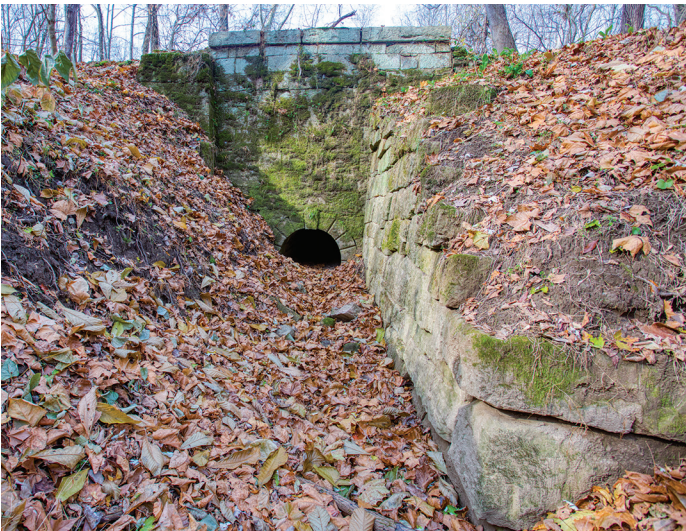
You may have noticed coping stones along the edge of the towpath as you traveled on Mile 132. They are the top of the high head-wall for Culvert 197, which features a long 90 degree wing wall on the downstream side of the outflow. An occasional stream flows through this 4-foot culvert. Photo by Steve Dean
