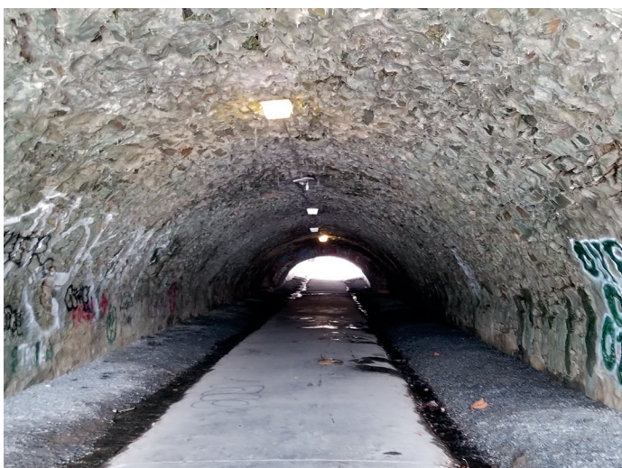
Foundry Branch Culvert barrel
