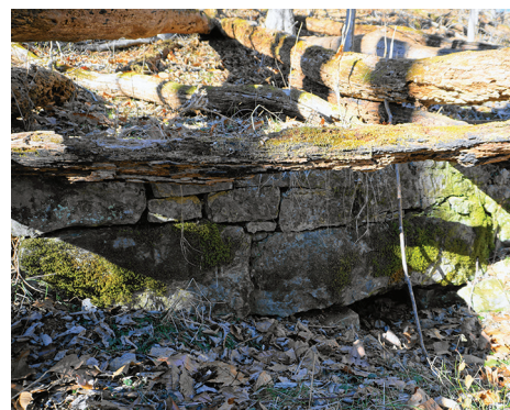
Buried box culvert
