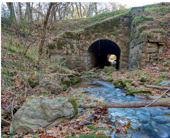
Culvert 192, at Mile 130, is located just above Lock 53 near Cohill Station. The 10-foot span culvert was built as a road culvert and now carries an active stream. The berm arch, shown here, requires a trek through briars but presents a striking view as the stream rushes over its rocky bed approaching the culvert. Photo by Steve Dean.
