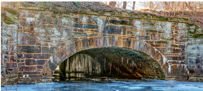
Culvert 93, at Mile 38, is located just above Lock 31 in Weverton. Israel Creek flows through its elliptical arch. The culvert is intact, but the berm breached over the berm in 2018. The towpath arch is above and the berm arch below. Ice often formed in the culvert barrel before the breach. Photos by Steve Dean.
