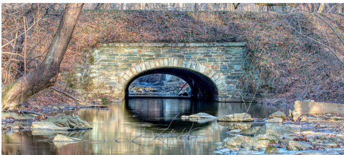
Culvert 93, at Mile 38, is located just above Lock 31 in Weverton. Israel Creek flows through its elliptical arch. The culvert is intact, but the berm breached over the berm in 2018. The towpath arch is above and the berm arch below. Ice often formed in the culvert barrel before the breach. Photos by Steve Dean.
