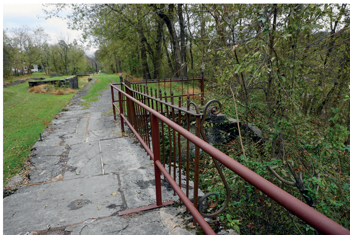
Below – Some of the original wrought iron railing can be observed on both ends of the aqueduct
