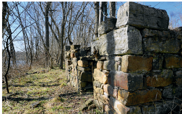
The beautiful stone work on the back basement door of the house near Locks 51 and 52. The mix of red shale and limestone blocks used to construct the house.
