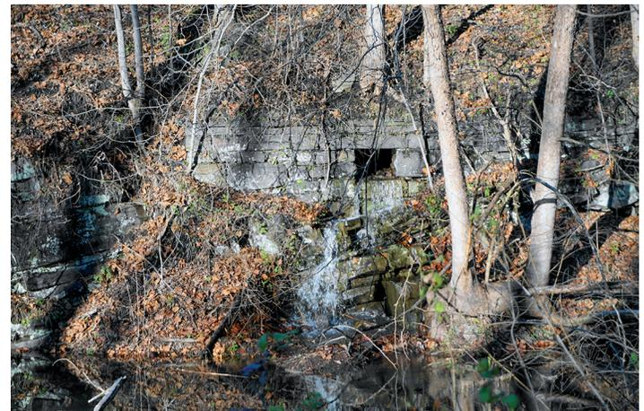
*A box culvert under the abandoned Western Maryland Railway right-of-way in the Town Creek area. It drains into the C&O Canal.*
