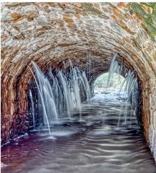
*Culvert 185, at Mile 126.42, is a 10-foot span sandstone culvert with a 5-foot rise. Also called Johnson's Culvert, it was built in 1836-1837. The stream is moderately active. When the prism above the culvert is watered the barrel leaks through numerous holes, creating a car wash effect. Upper – berm arch; side – barrel; lower – towpath arch.
