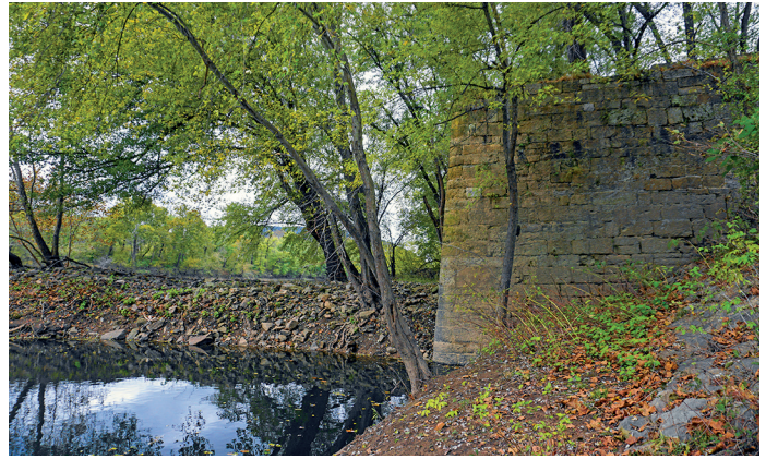
The remains of Dam 6.
