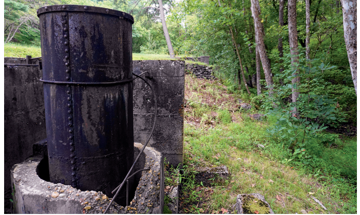
Creosote (wood preservative) dipping tank at Lock 66.
