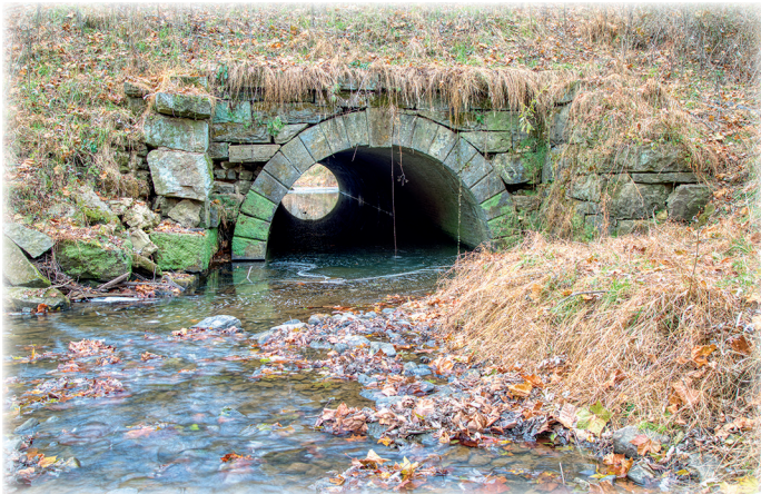
Culvert 231 is at Mile 173.8, just above Spring Gap. It is a 12-foot span culvert and carries Collier Run under the canal. Like many Western Maryland culverts, it is brick lined. Around 84,250 bricks were used in its construction. Above – towpath arch. Below – berm arch. Photos by Steven Dean
