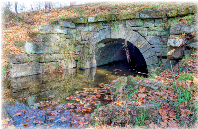
Culvert 231 is at Mile 173.8, just above Spring Gap. It is a 12-foot span culvert and carries Collier Run under the canal. Like many Western Maryland culverts, it is brick lined. Around 84,250 bricks were used in its construction. Above – towpath arch. Below – berm arch. Photos by Steven Dean
