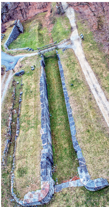
Lock 38 overhead view from the Rumsey Bridge. The extension of the lock can be seen in the upper part of the photo, along with the abutments of the old road bridge at the upper end of the extension. The bypass flume is visible on the left, with a buried culvert under the crossover. For further information about Lock 38, refer to the Towpath Guide to the C&O Canal by Thomas Hahn.
