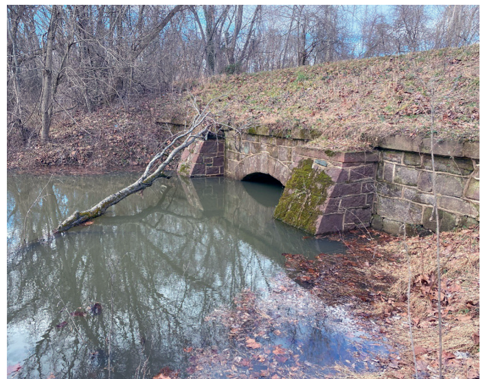
High water at Culvert 72 – Photo by Bob Carpenter
