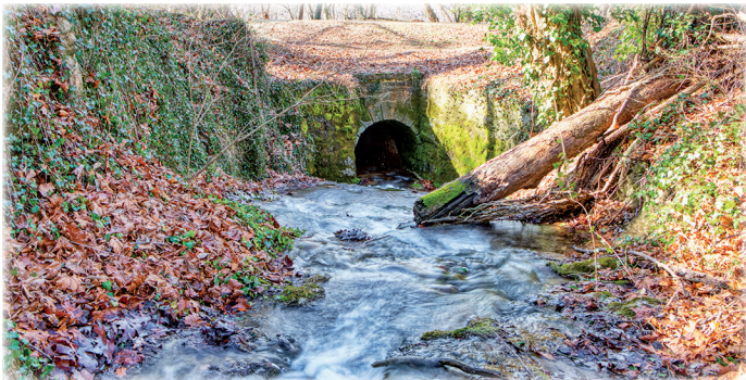
Long- and medium-hikers in the Douglas Hike will cross Culvert 115, the Mondell Culvert, at Mile 80.55. This 6-foot culvert carries an active stream with rapidly flowing water over a rock stream bed. The outflow (above) leads directly into the Potomac River. The inflow stream (left and below) flows down hill into the culvert. Hikers can cross the prism to view the inflow stream. Photos by Steven Dean
