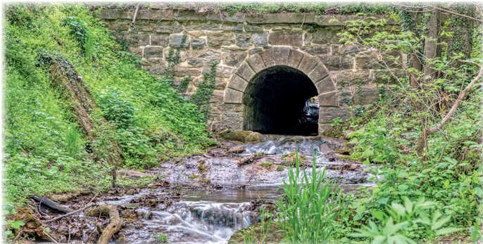
Long- and medium-hikers in the Douglas Hike will cross Culvert 115, the Mondell Culvert, at Mile 80.55. This 6-foot culvert carries an active stream with rapidly flowing water over a rock stream bed. The outflow (above) leads directly into the Potomac River. The inflow stream (left and below) flows down hill into the culvert. Hikers can cross the prism to view the inflow stream. Photos by Steven Dean
