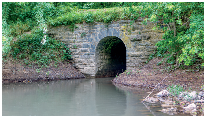
Culvert 116 – Marsh Run Culvert
