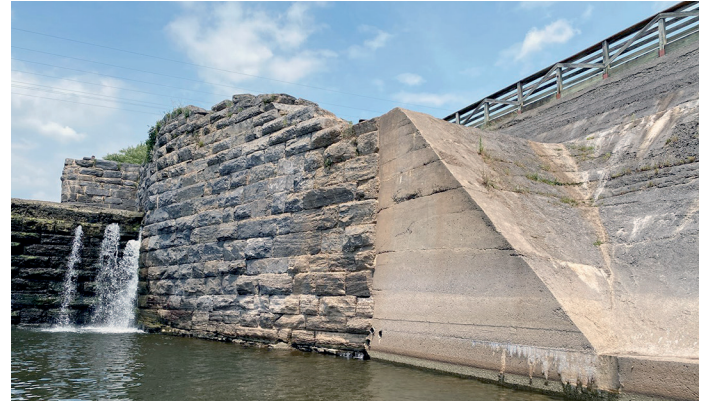
Dam 5 left abutment detail
