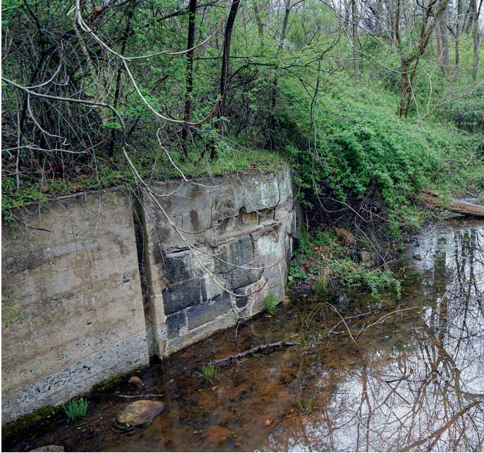
A view of the Big Pool western stop gate plank slot
