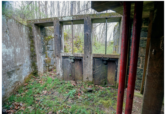
Butterfly gates in the waste weir above Lock 50 at Four Locks
