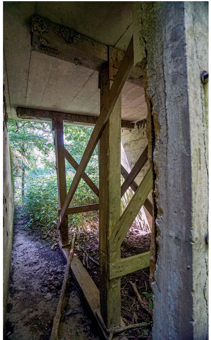
Detail of timber cribbing supporting a waste weir bridge
