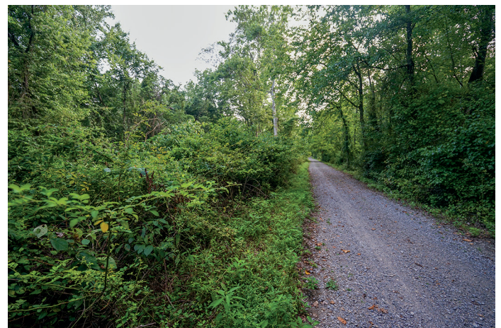
Hedges tend to send out limbs that extend out into the towpath and interfere with the travel path. This area was cut by park maintenance a few weeks prior using a mechanized scythe blade mounted on a tractor.
