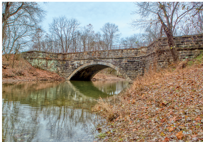
Town Creek Aqueduct – Photo by Steven Dean
