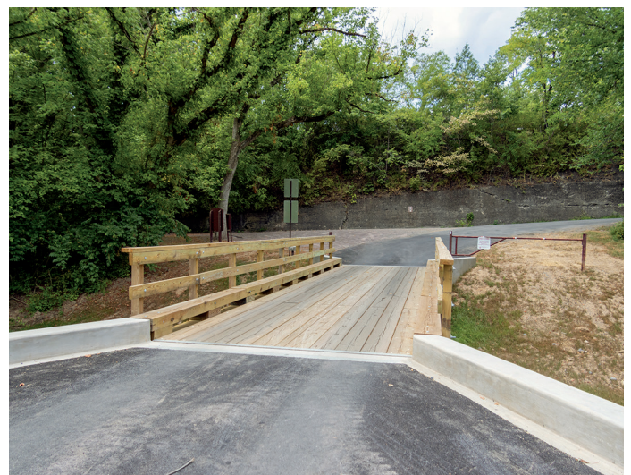
Crossover bridge at Fifteen Mile Creek – Photo by Steven Dean
