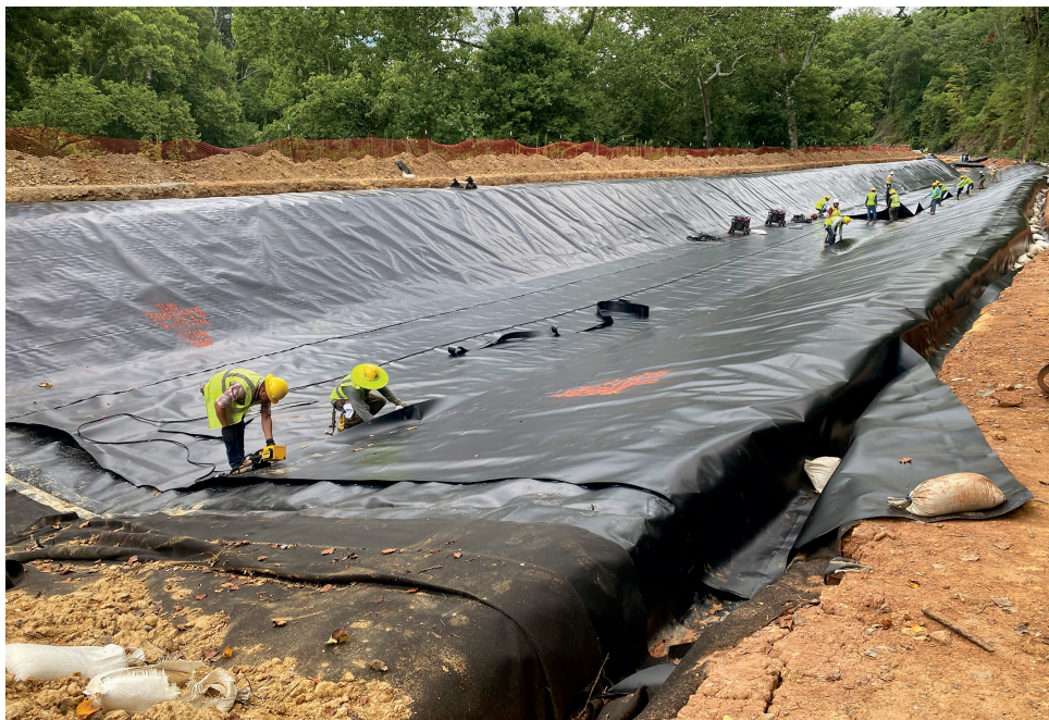
The installation of the canal prism liner – Photo by C&O Canal Professional Services Division
