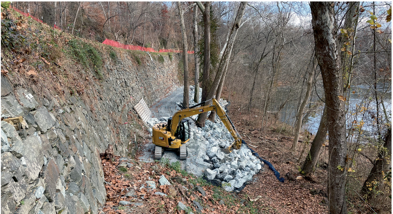
The building of the Log Wall upstream riprap buttress – Photo by C&O Canal NHP Professional Services Division
