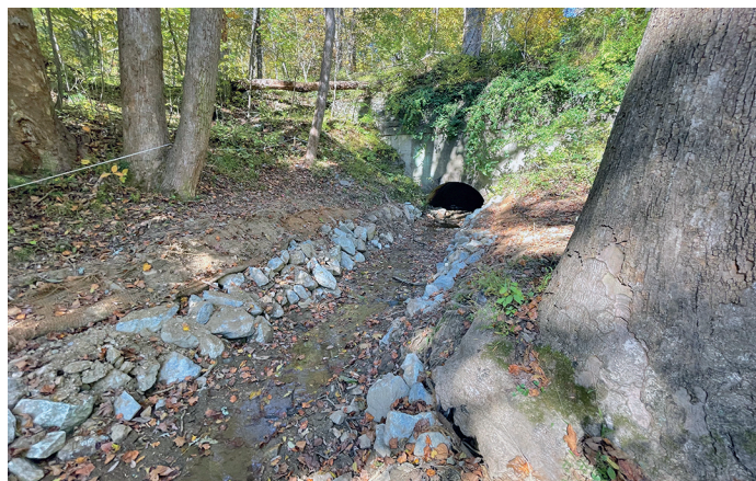
The stabilization of a tributary leading into the canal prism – Photo by C&O Canal Professional Services Division
