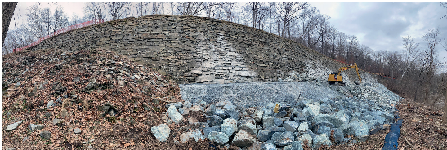
Panorama view of the construction of the upstream buttress – Photo by C&O Canal Professional Services Division
