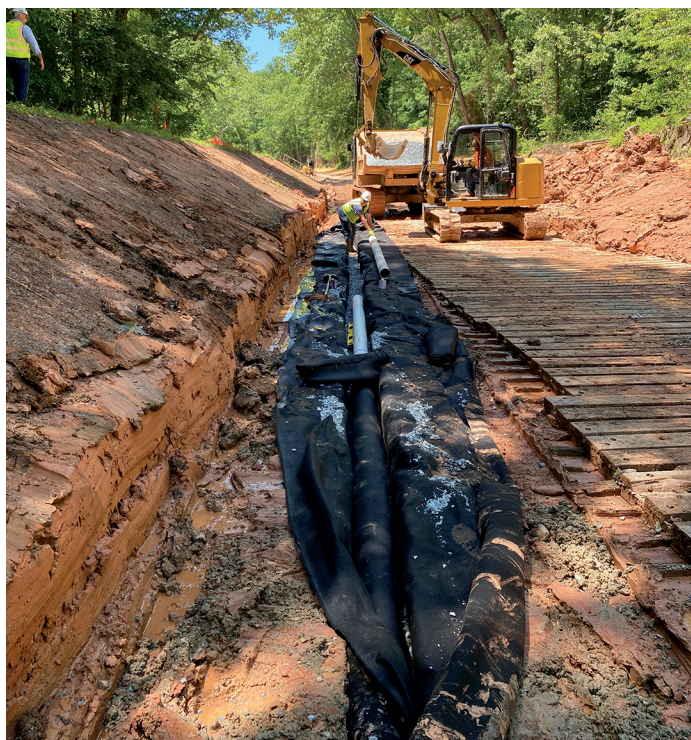
The installation of an underdrain system within the canal prism – Photo by C&O Canal Professional Services Division
