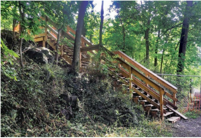
Stairway at detour around Dam 5 construction.
