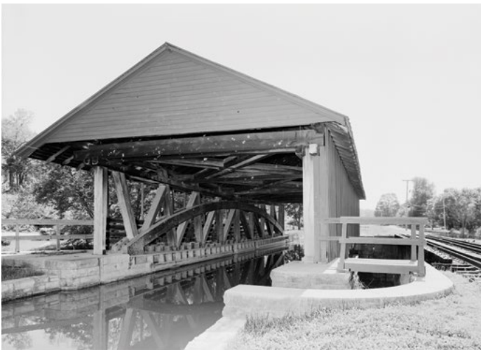
(Above) Duck Creek Aqueduct, Metamora Indiana. Photo courtesy Library of Congress. (Right) Wabash and Erie Canal Park, Delphi, Indiana. Photo by Robert Schmidt
