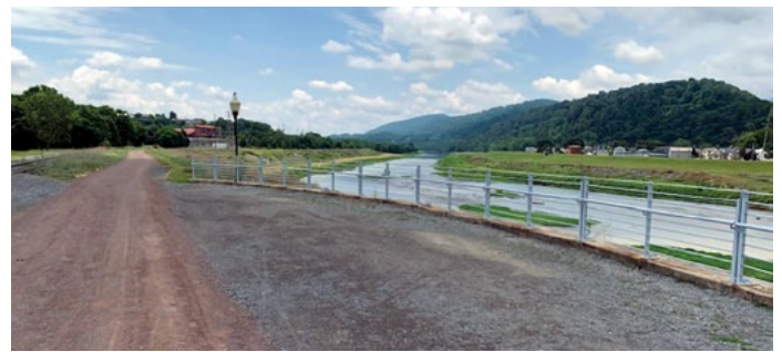
Towpath resurfacing in Cumberland. Photo by Travis Medcalf
