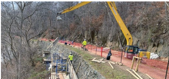
(Top to bottom) The Log Wall at Mile 11 (a dry-laid stone wall nearly 200 years old) before repairs, during construction, and after completion in June 2025. Photos courtesy NPS
