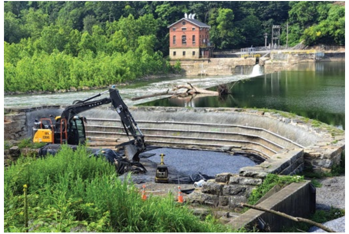
Abutment at Dam 5 will be filled with dirt.
